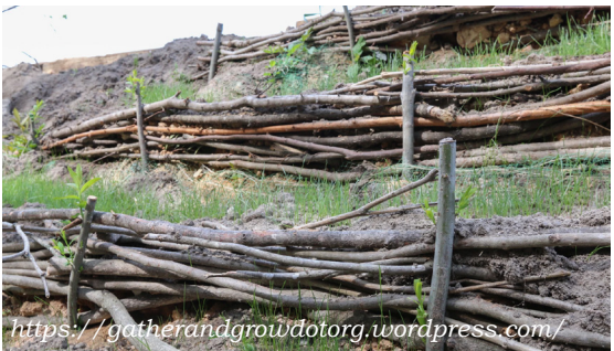
A wattle retaining fence staked with live tree cuttings that simultaneously revegetates and builds soil is one approach to stabilizing slopes.
