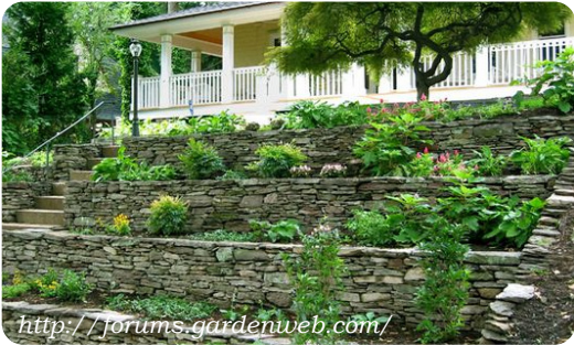
Vegetated retaining wall terraces slow and sink water and the lower beds are at a height that makes harvesting easier from a seated position or without bending down.
